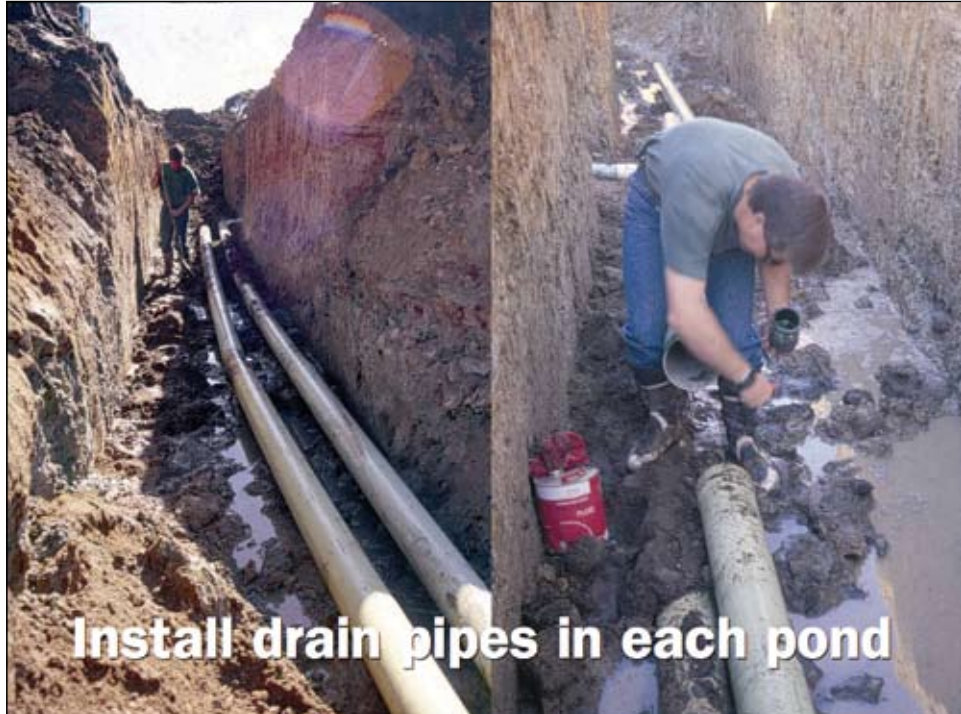
Slide 12. Install drain pipes in each pond.
