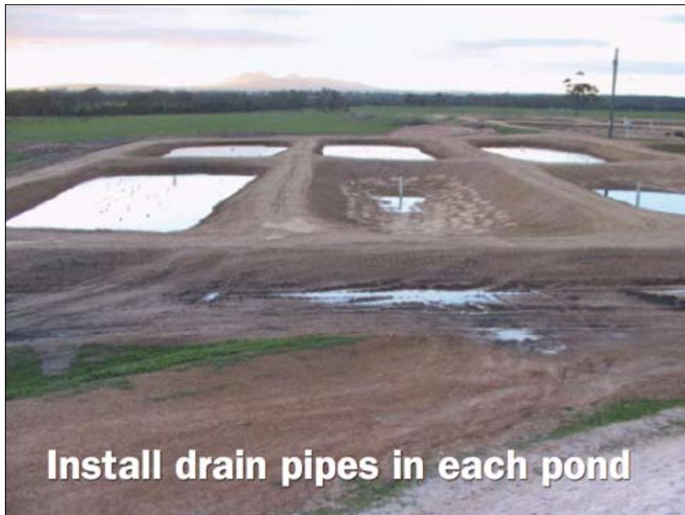
Slide 13. Install drain pipes in each pond.
