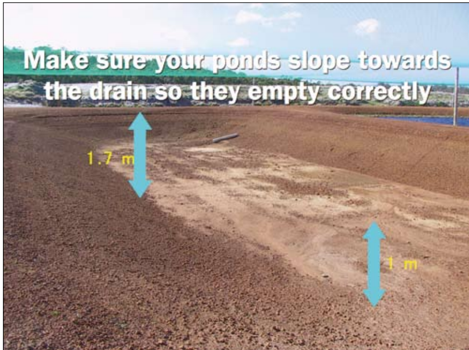
Slide 16. Make sure your ponds slope towards the drain so they empty correctly.
