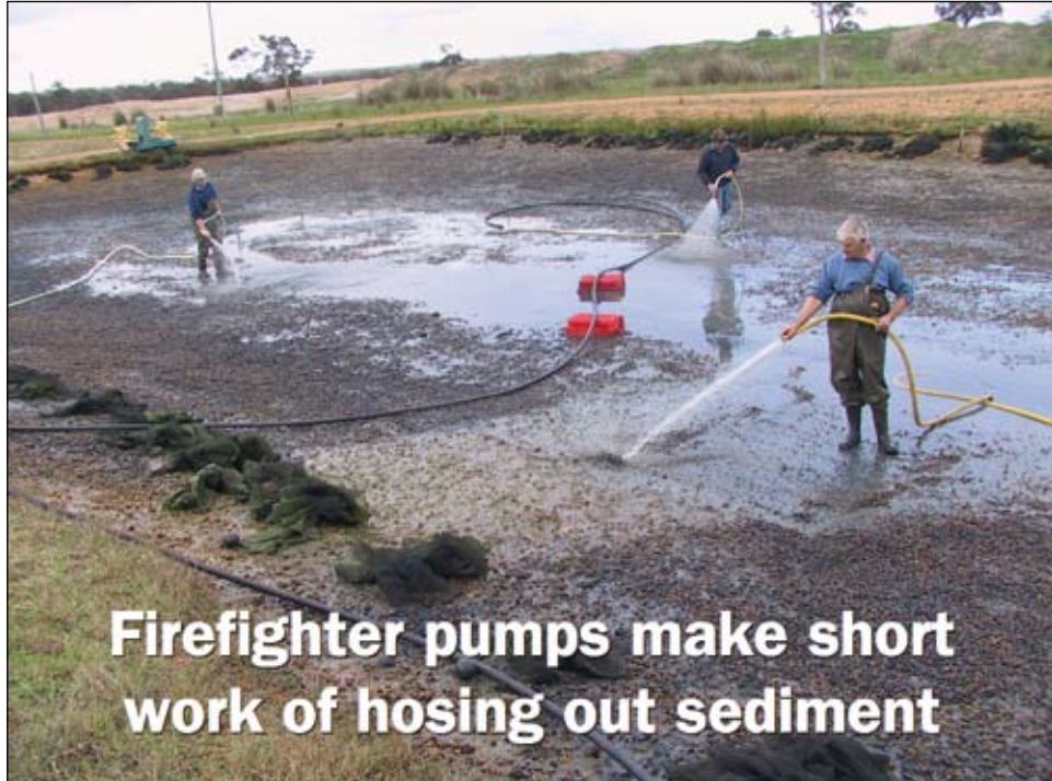
Slide 45. Firefighter pumps make short work of hosing out sediment.
